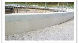
**The outcome:** The concrete walls to the two PSTs were successfully re-profiled, with the tops of the walls provided with a level running surface with an anti-slip finish as had been desired by the Client (YW). The protective coating system added increased durability to the repaired wall
