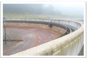
**The solution:** Reforming and maintaining the original profile to the tops of the walls was of paramount importance due to the alignment requirements of the running wheel to enable the agitator boom to run around the circumference of the tanks all year round as well as the obvious loading and wear resistance associated with it. **APA Concrete Repairs Ltd** devised a programme of repair and protection works that included the installation of fixed scaffolding
